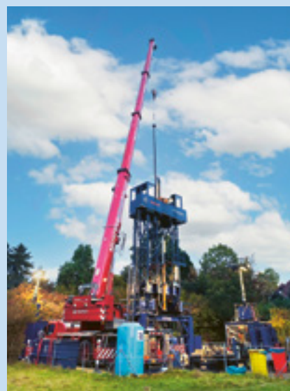
Complex rehabilitation operation with snubbing unit in Switzerland. © CFG
