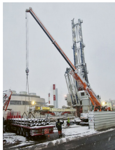
Drilling for the installation of geothermal doublets at Roissy. © CFG GÉOTHERMAL
