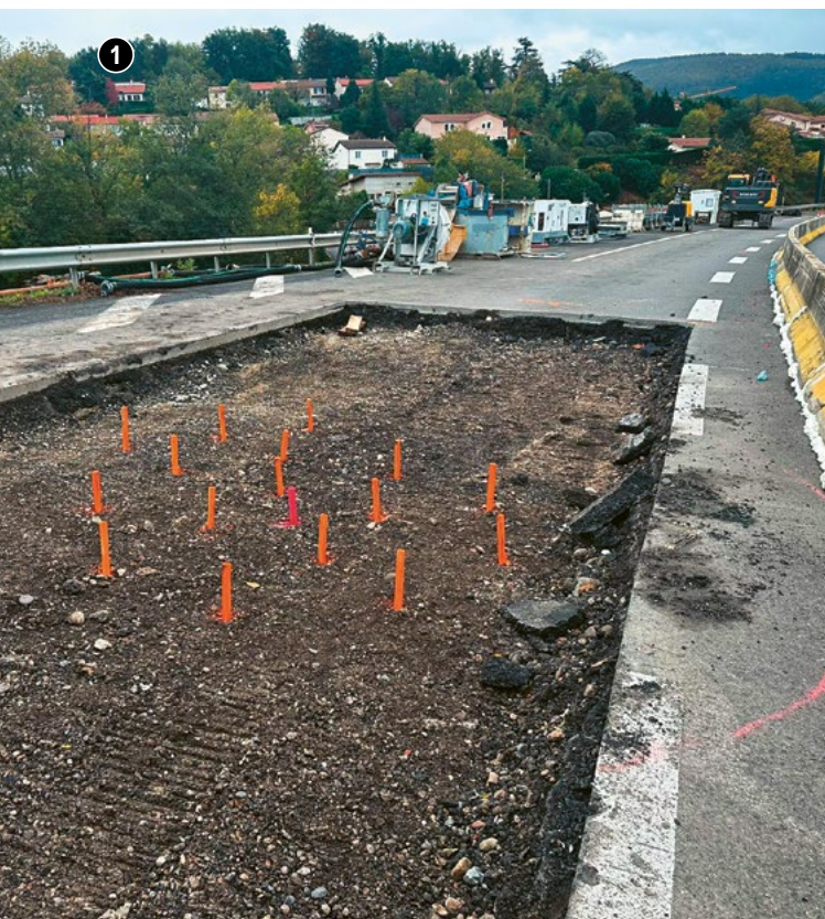
1 Installation of jet grouting columns in the backfill of the former mine shaft located beneath the Saint-Étienne motorway bypass. © BRGM
